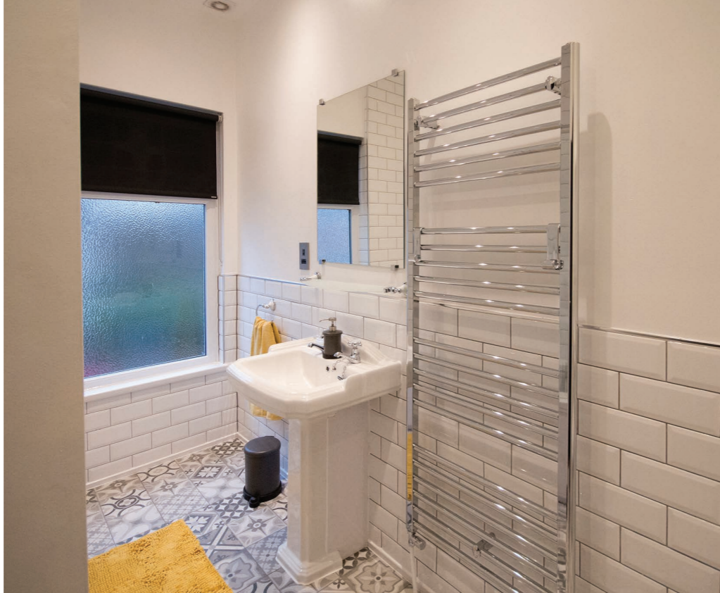
The same corner – refurb completed
