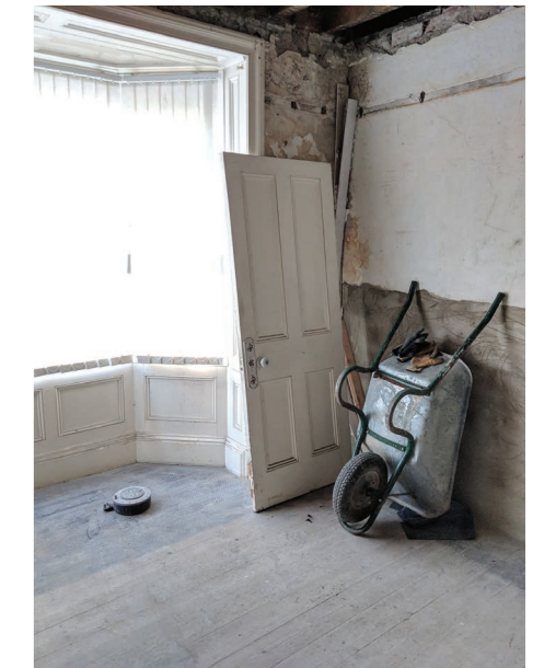
Tanking completed to the affected walls (scuse the door and wheelbarrow!)
