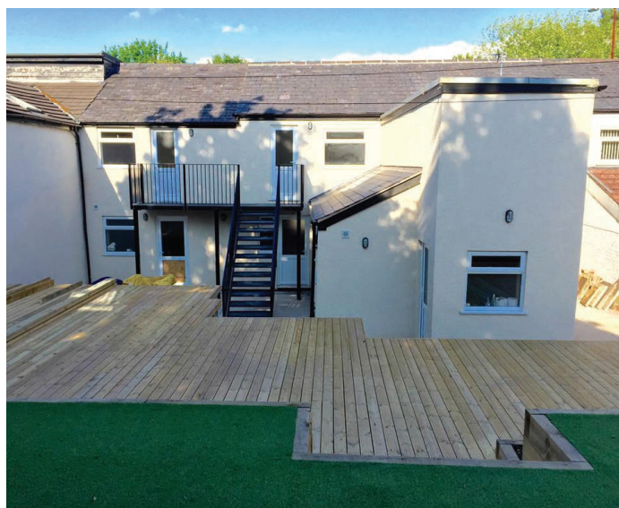
Large communal sociable space, with secured access, to the rear of ten one-bed apartments in Dukinfield, Tameside
