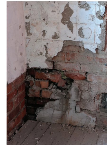
Additional structural works uncovered when peeling back the layers
