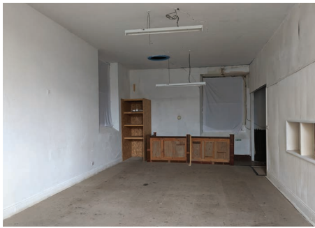
A side room on the first floor
