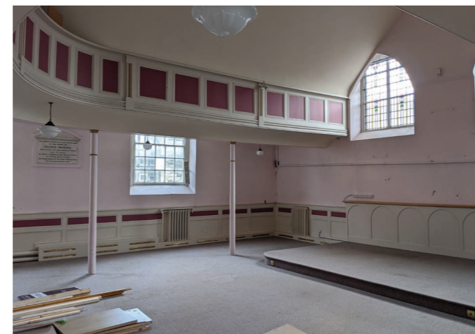
The existing balcony area, with poles which must be retained
