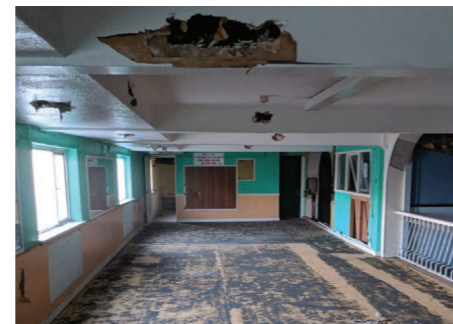
First-floor outer area at the start of the project
