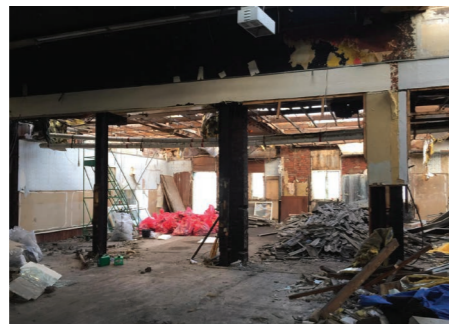
Ground-floor central area as the work commenced
