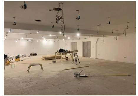
The central conference area nearing completion
