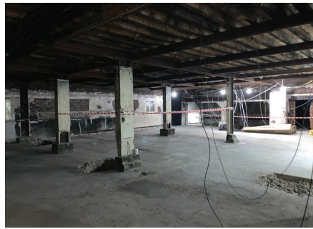
Ground-floor central area under development
