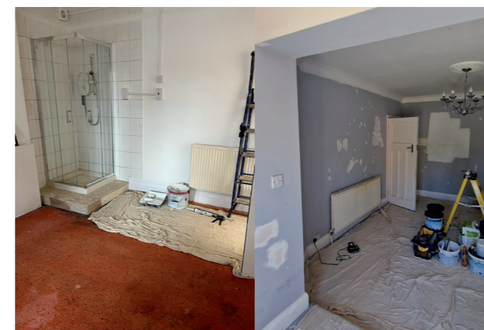
One of Athena's properties under refurbishment
